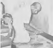
A MECHANICAL Department carpenter puts the finishing touches on the newly-laid out offices, above. Moving in, below, is Rudy Yzer, head of housing maintenance and renovation.
